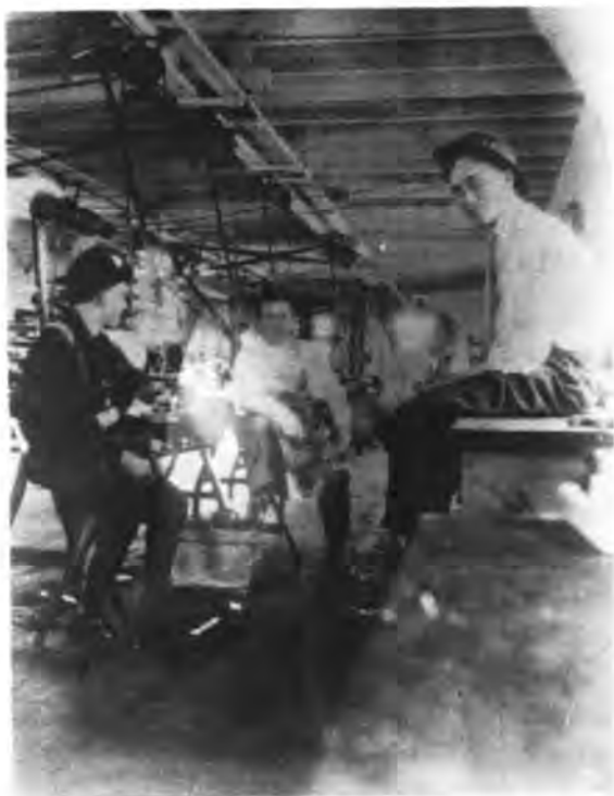
United Wireless Telegraph Company's Machine Shop At Seattle, Washington. Right Eden Haw. Photo by: Gordon Haw
